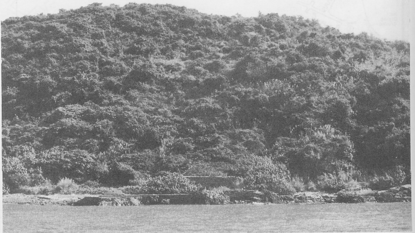
Plate 4 The stone building in the southwestern corner of the island, which used to serve as the ore bin, still survives, as does the nearby jetty from which the graphite ore was loaded onto sampans
